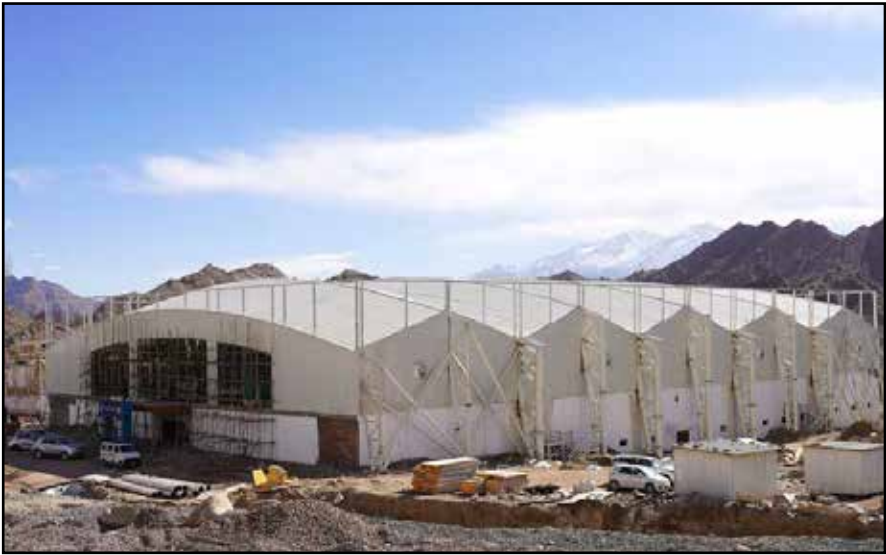
Photo Caption: Under construction international-standard indoor ice hockey rink at NDS Stadium, Leh. Reach Ladakh Correspondent
