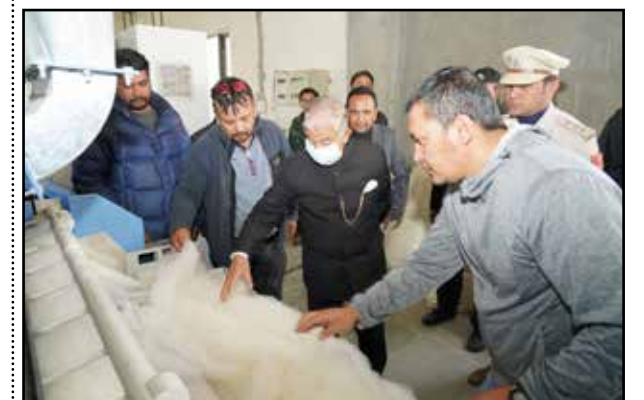
Lieutenant Governor of Ladakh, Brigadier (Dr) BD Mishra (Retd) inspecting the newly installed Pashmina Dehairing Plant at the Industrial Estate in Leh.
