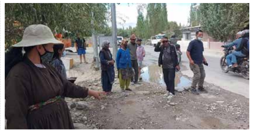
Residents of Agling village expressing frustration over the malfunctioning of the Sewage Treatment Plant (STP).
