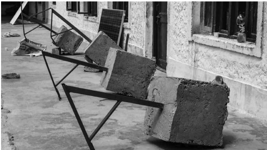
Fallen cemented blocks to hold solar panel due to strong wind at Shey Lamdon.
